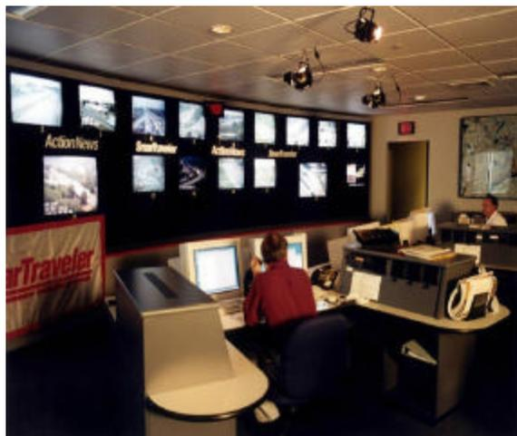
Figure 1: Intelligent Transportation System control facility.
