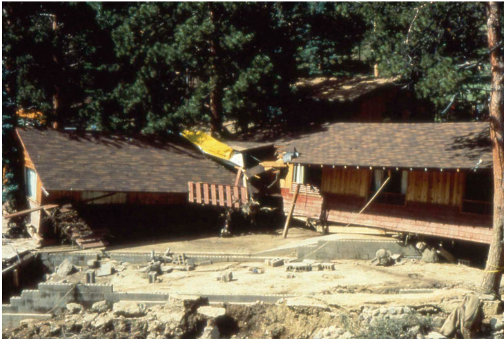
Photograph of building moved off foundation by flash flood.
