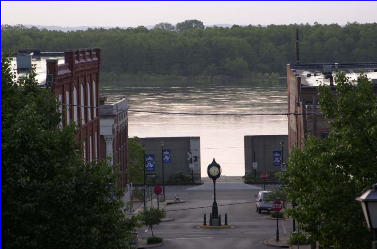
A levee on the Mississippi River in Missouri. (Source: FEMA)
